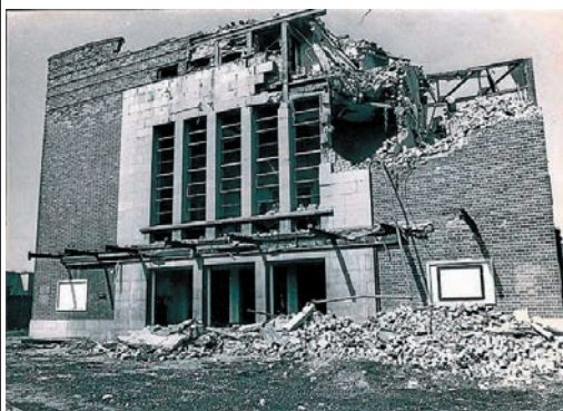
End of an era...the demolition of the Penn Cinema in 1973. Photo Nigel Caddick.
